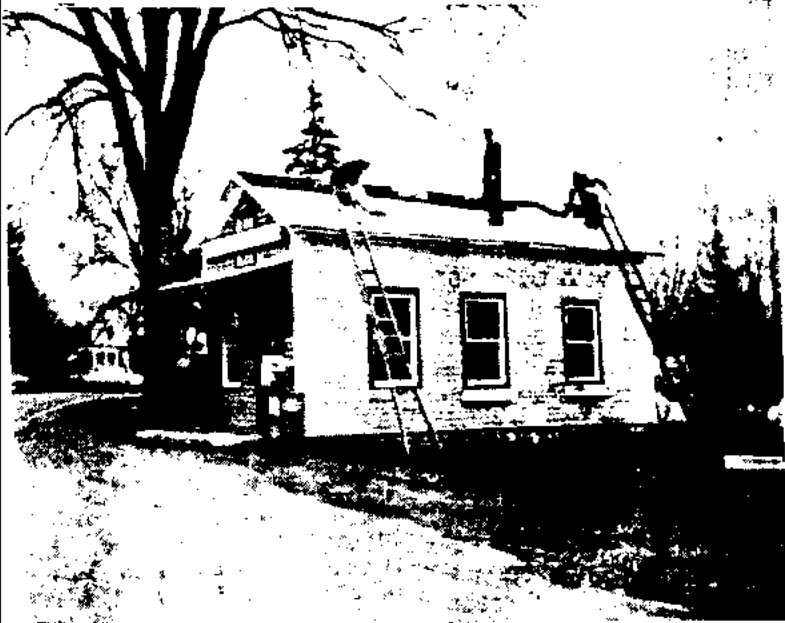
Post Office Roof Project
